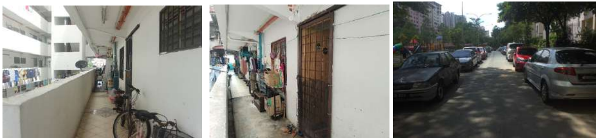
Figure 6. Issues related to obstruction of thoroughfare at PPR Kerinchi
