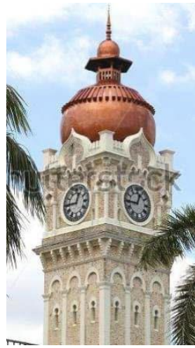
Figure 5. The onion dome of the clock tower is crowned by a domed-chhatri.
