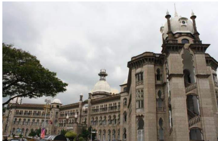
Figure 17. View of the railway administration building.
