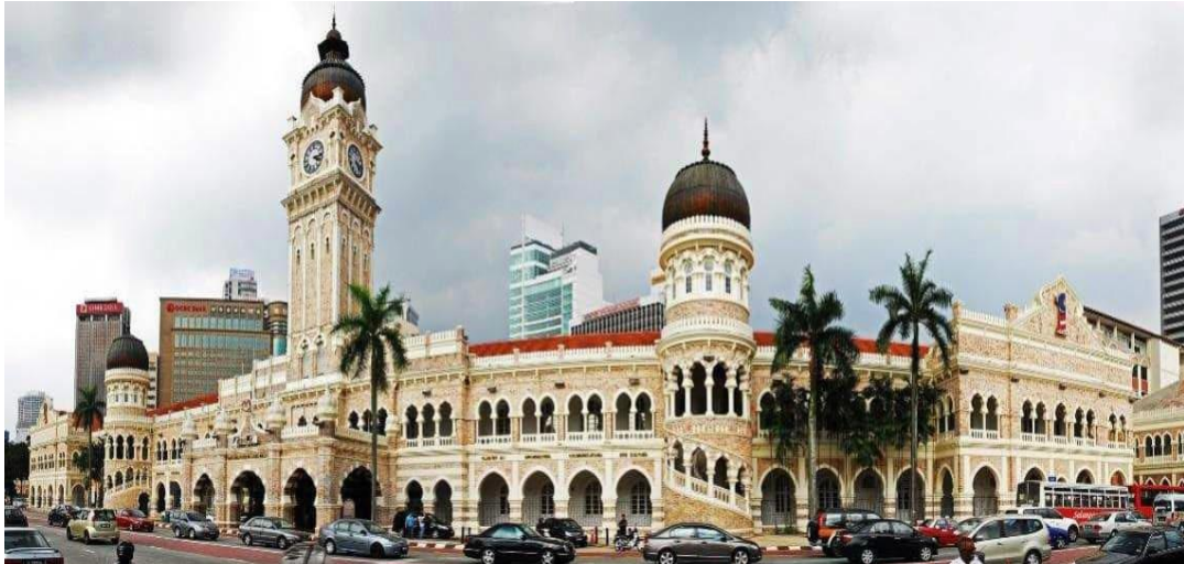
Figure 2. Sultan Abdul Samad Building.
