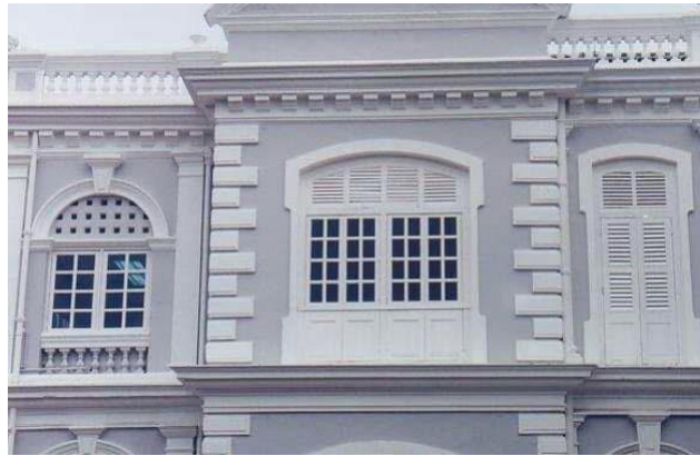
Figure 13. Plaster renderings at cornices, mouldings and front parapet wall (Ahmad 2004).
