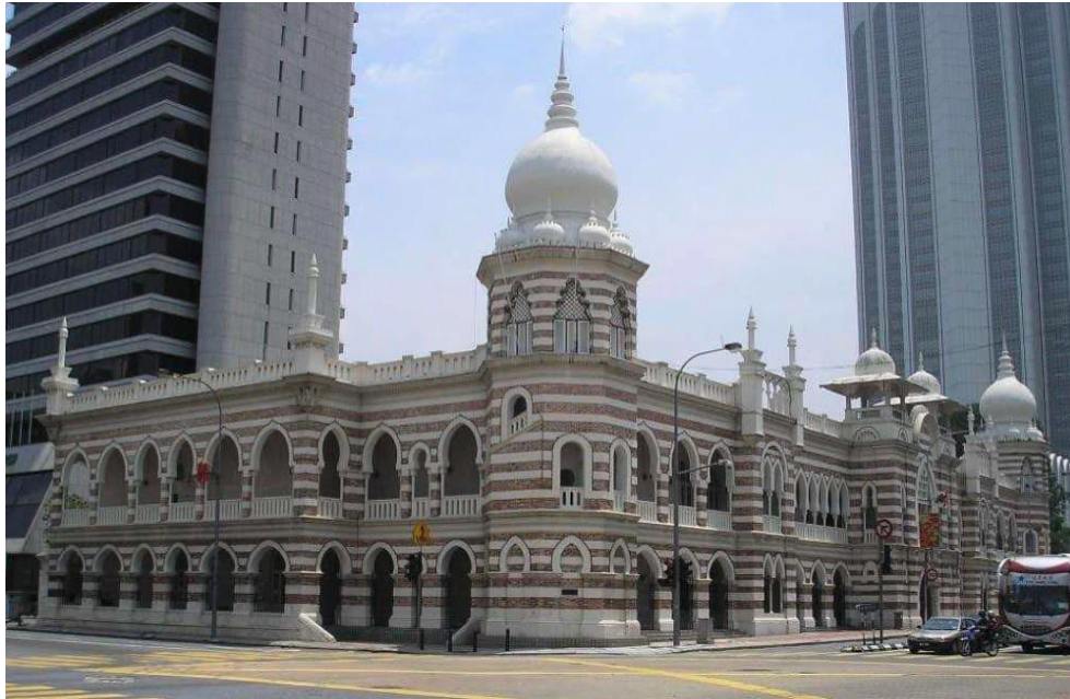
Figure 7. View of Old Public Works Department (Fieldwork 2010).
